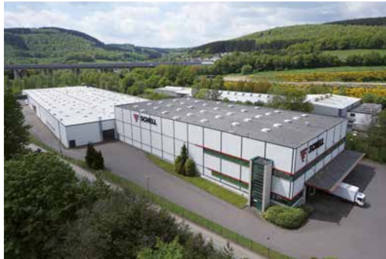
Plant 2 Production with logistics centre
