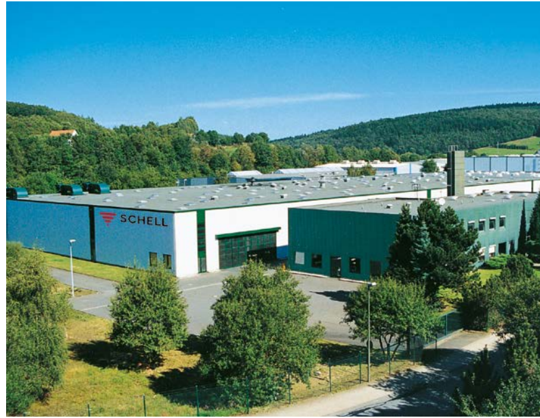
Plant 2 Production with logistics centre
