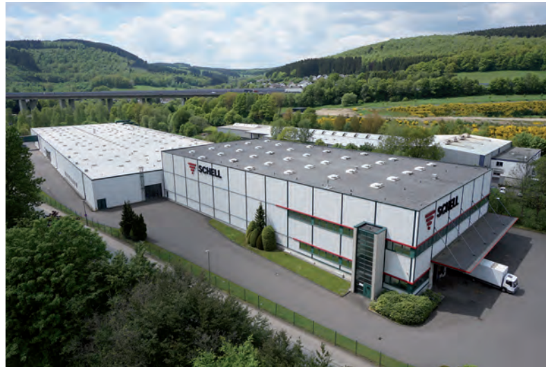
Plant 2 Production with logistics centre
